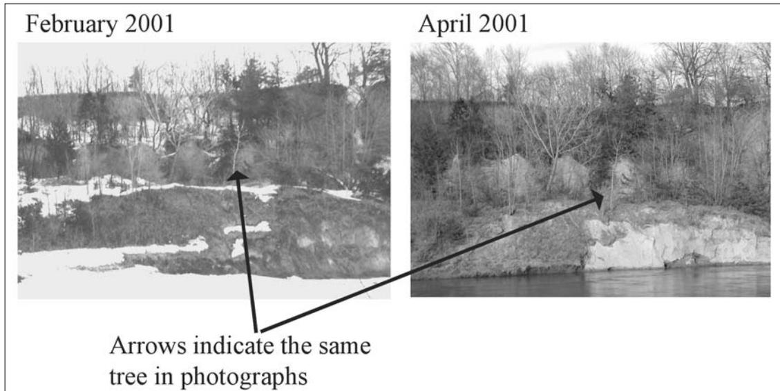
Figure 2. Two views of a bank along the Blue Earth River showing the occurrence of seasonal erosion. The light colored area in the lower right of April 2001 image is where some sloughing has occurred since February 2001.
