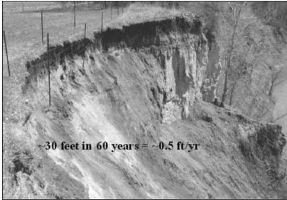
Figure 1. A view of the bank sloughing along the Blue Earth River. Hanging fence showing the recent failure in the top portion of the bank. According to owner of this field, the banks have receded about 30 feet in his lifetime (60 years) giving bank erosion rate of 0.5 ft/year.
